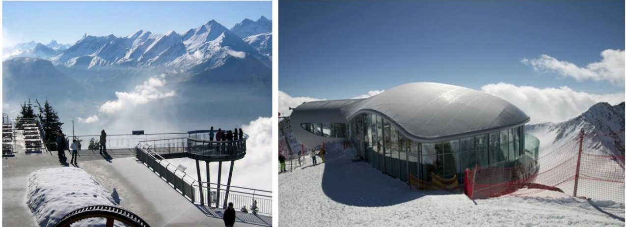
Figure 19: Representational images of a viewing deck and chair-car lift (ski-lift) terminal station
