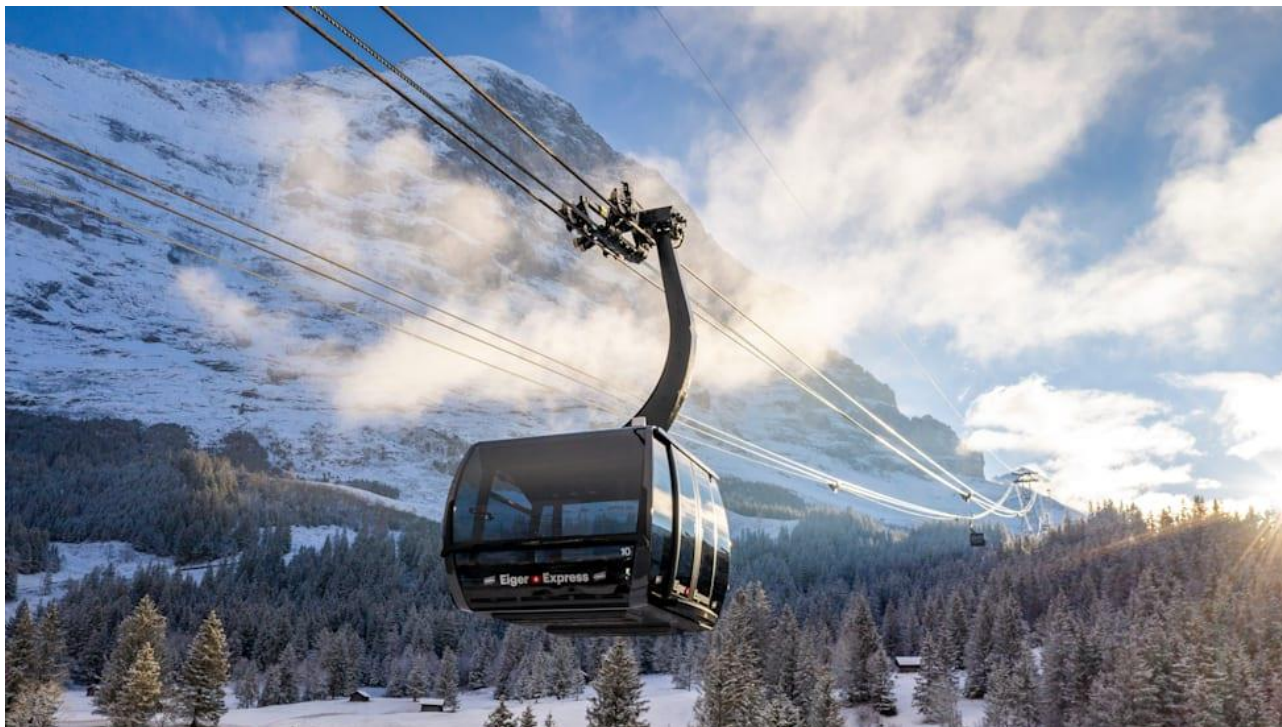
Figure 21: 3S / Tricable Ropeway System/Aerial Tramway
